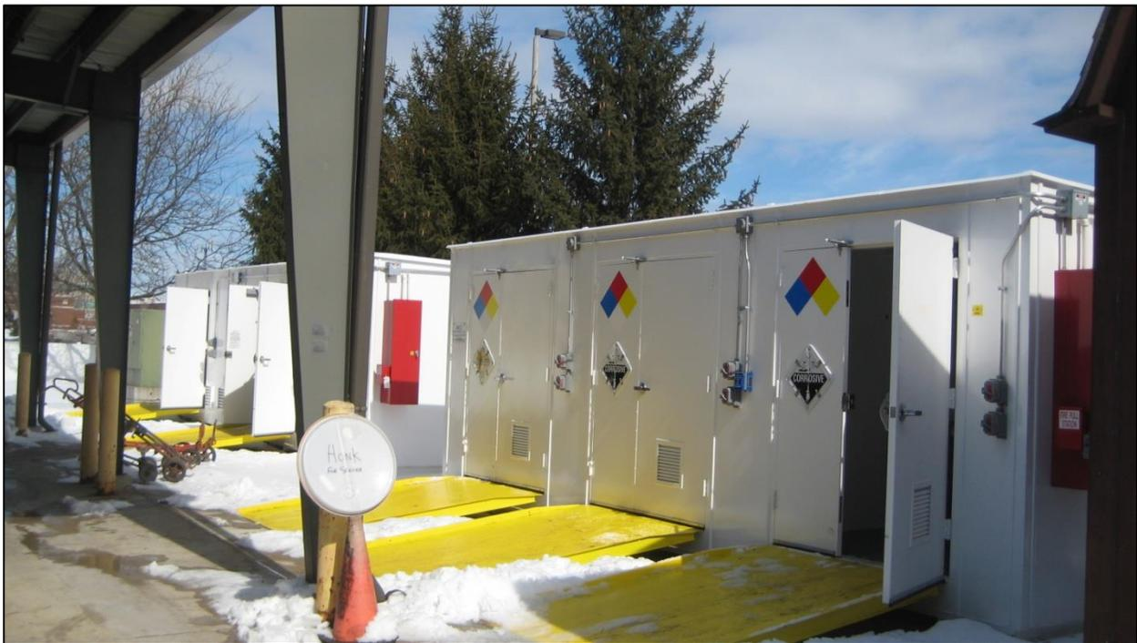
Figure A-2. Secured Prefabricated Hazardous Material Storage Units at Naperville Facility.
